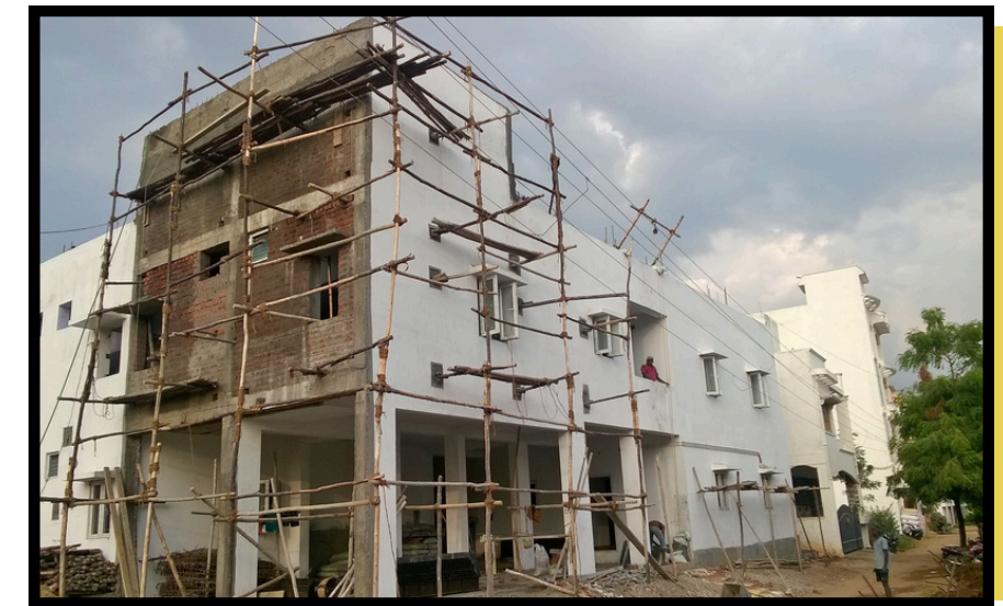
APARTMENT BUILDING ERODE
